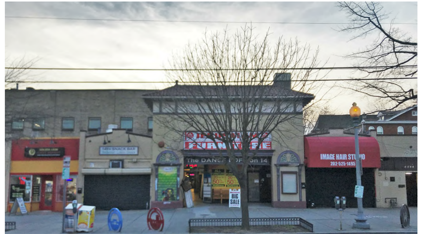
B. FURNITURE STORE FACADE
